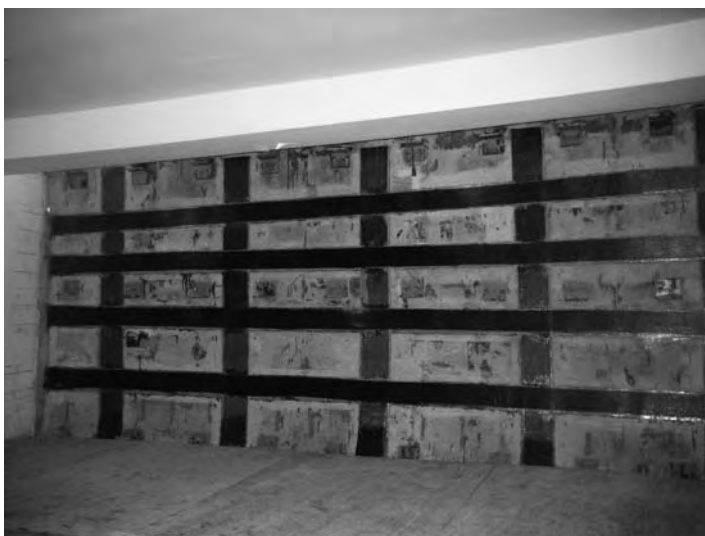
Figure 6 Carbon fibre reinforcement at the interior face of the Guggenheim Rotunda's uppermost wall (© A. Ayón, WASA/Studio A, 2007).
