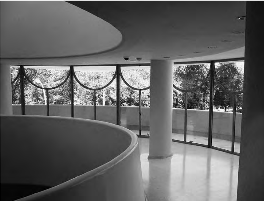
Figure 9 Replacement thermally broken steel-frame glass walls, 3rd Floor Thannhauser Gallery (© The Solomon R. Guggenheim Foundation, 2008).
