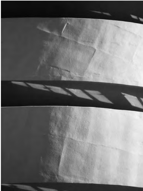
Figure 5 Detail of Rotunda wall showing original formwork marks after exterior conservation work (© A. Ayón, WASA/Studio A, 2009).
