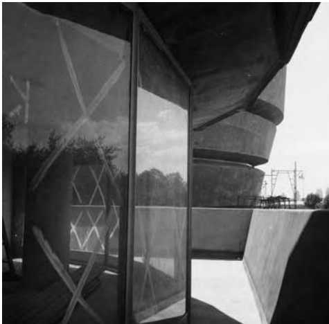
Figure 8 Frank Lloyd Wright, Solomon R. Guggenheim Museum, original steel-frame glass walls during construction (© William Short, the Solomon R. Guggenheim Foundation).
